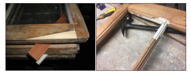
**Dutchman's:** Where signs of rot occur, it is important to remove the deteriorated section and install a dutchman. This can be done with wood or alternative materials such as epoxy.
