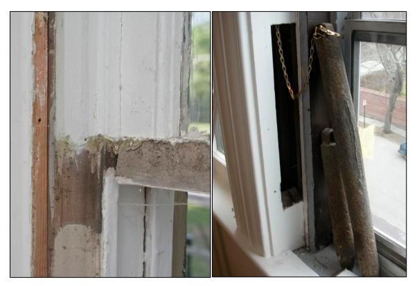
**Operation:** Cutting the paint seal while replacing the sash cords/chains will increase the functionality of your windows. Before and after example below.
