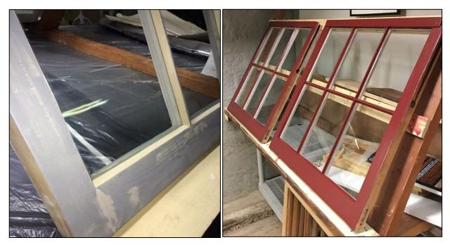
**Glazing Putty:** When you see signs of glazing putty failure, it is important to remove deteriorated sections and install new glazing putty and paint accordingly.
